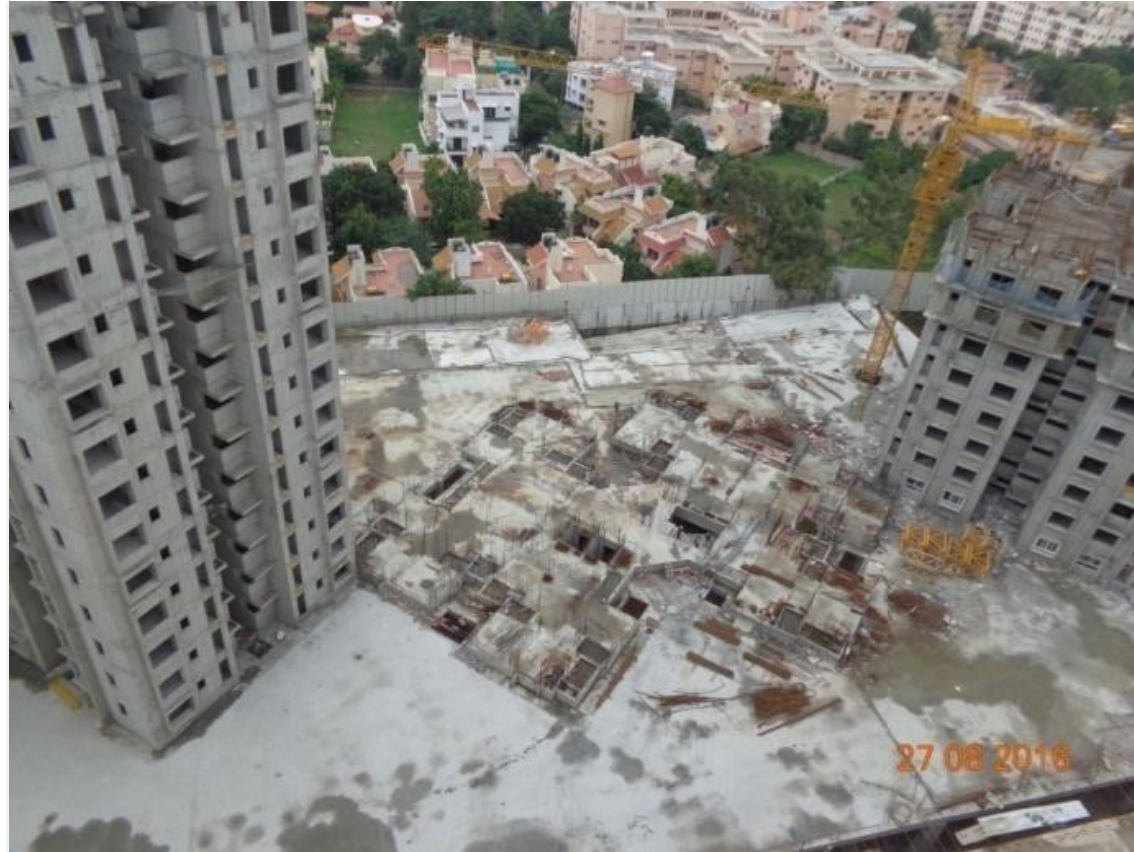
TOWER J Level 2 Work In Progress
