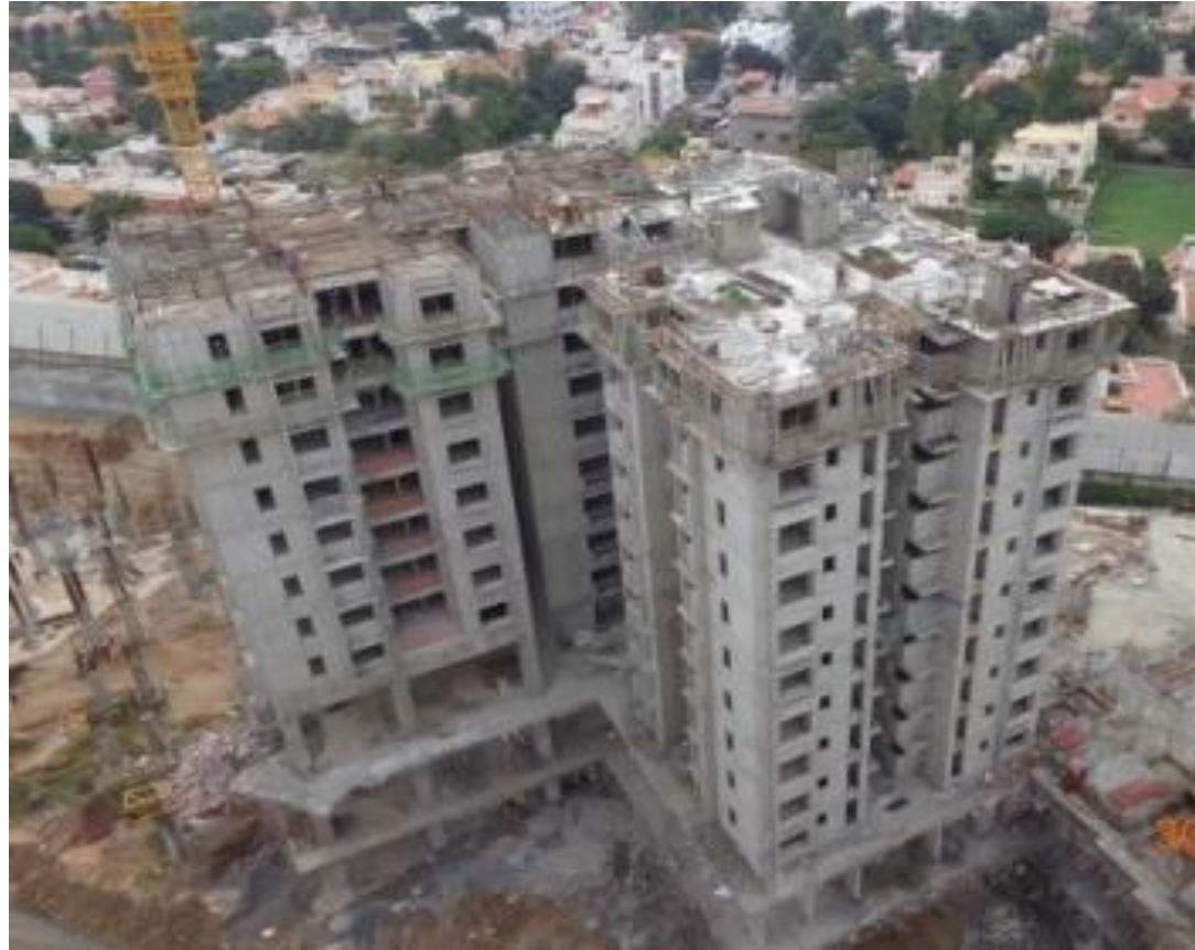
TOWER K : Level 10 Roof Completed
