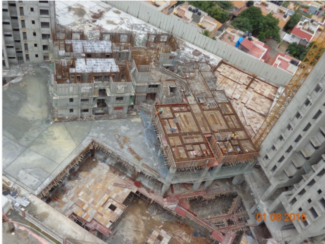
TOWER L Level 2 Work in Progress
