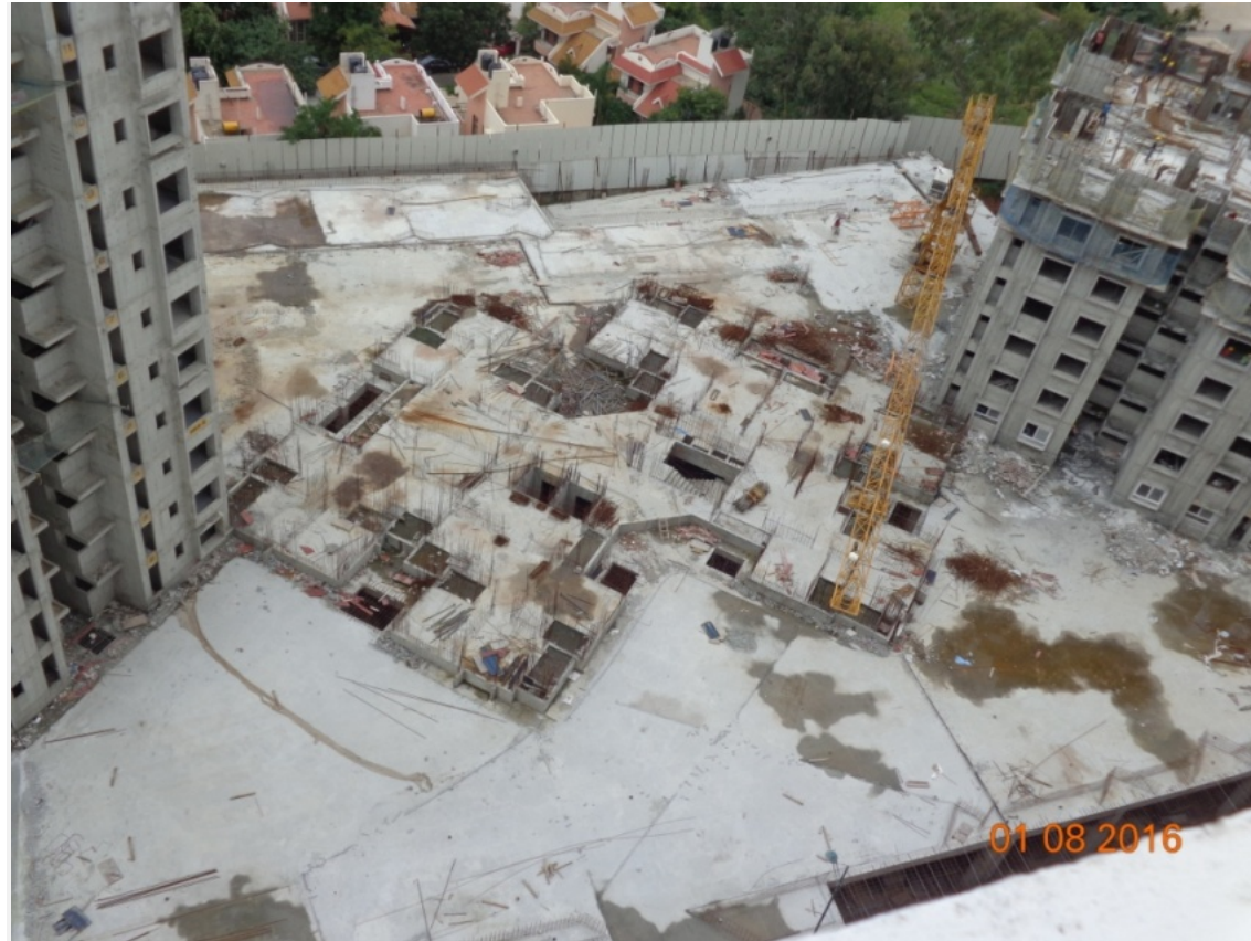
TOWER J Level 2 Work in Progress
