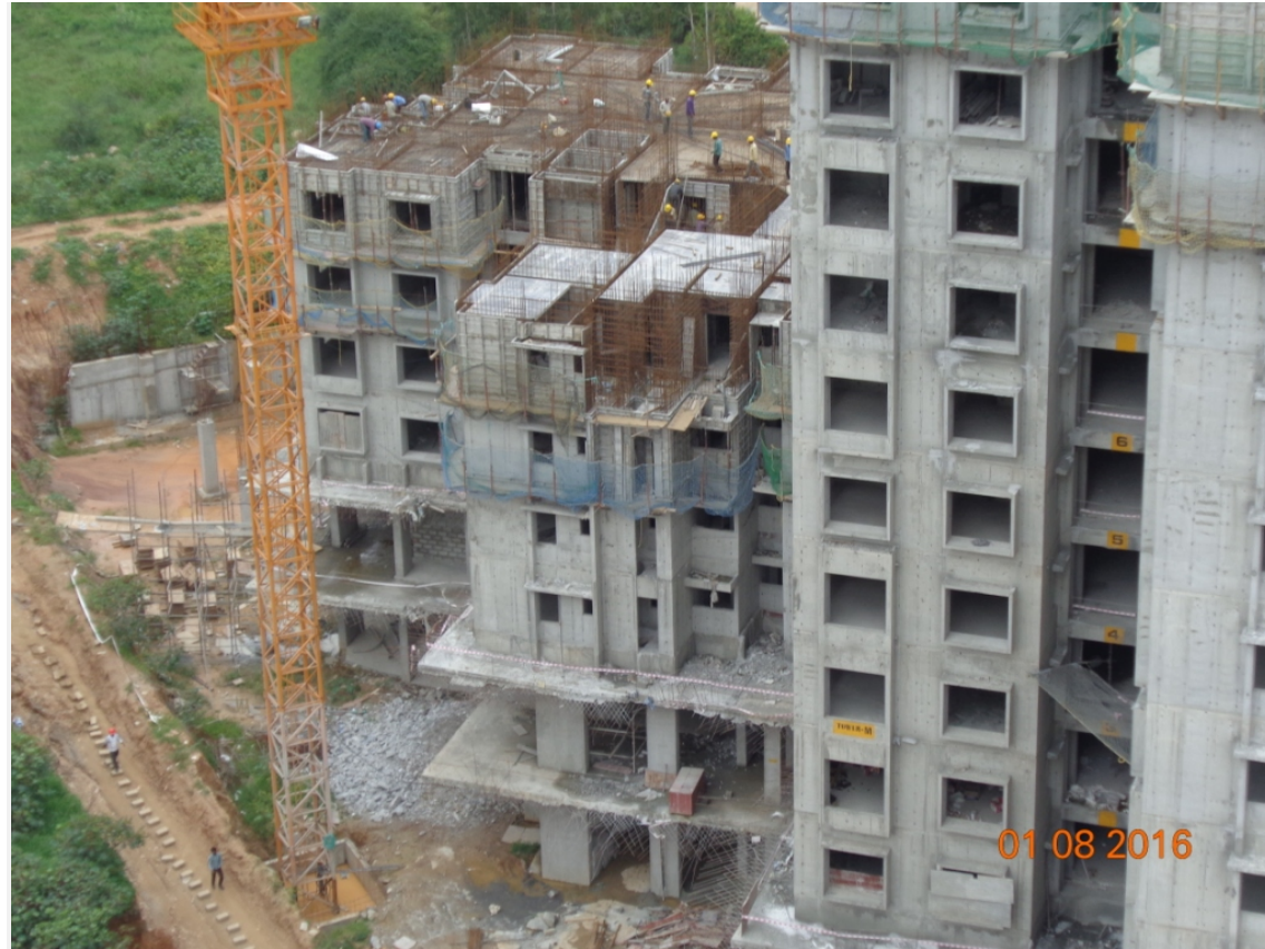
TOWER N Level 4 Roof Work in Progress
