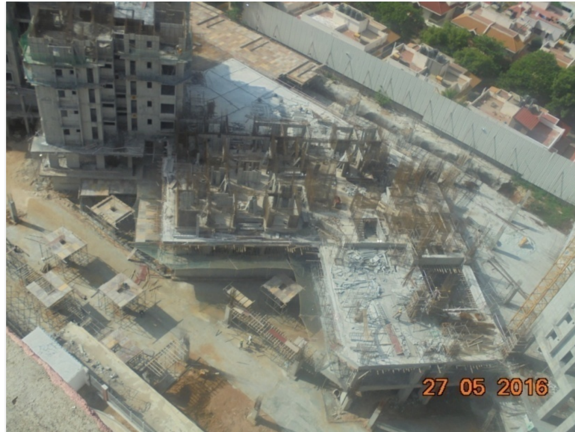
TOWER L Level 2 Work In Progress
