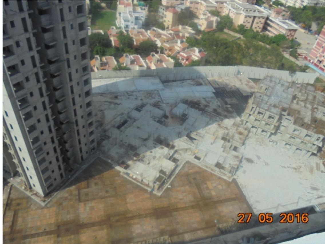
TOWER J Level 2 Work In Progress
